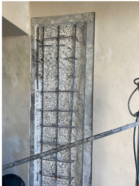
Picture 2: Completed excavation on the divider walls
