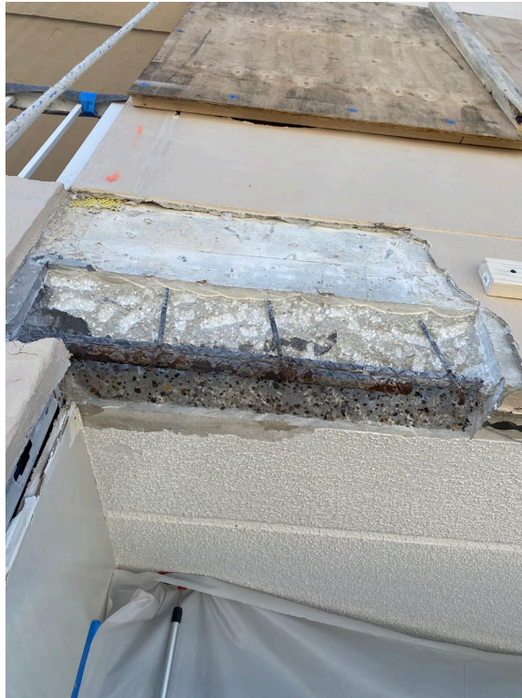
Picture 3: Header repair at Unit 505
