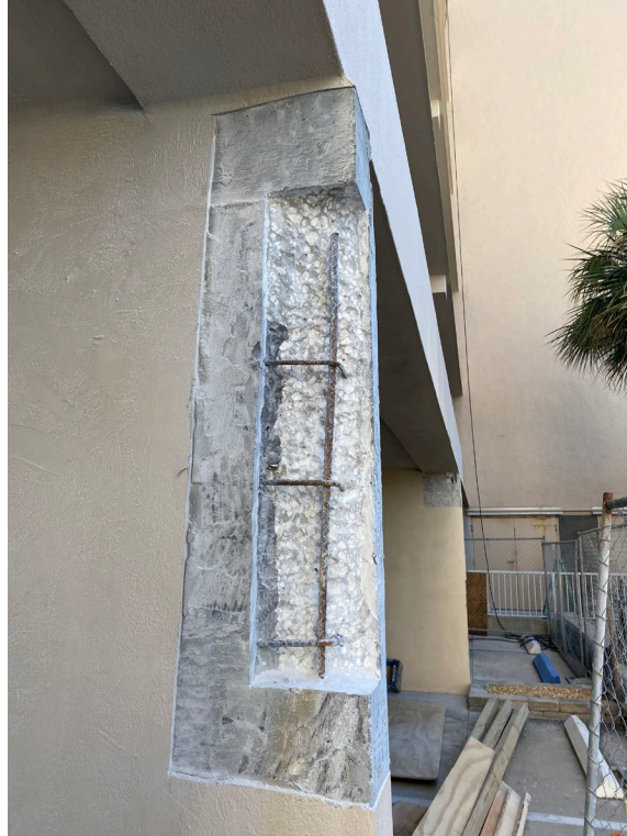
Picture 1: Completed excavation on the divider walls
